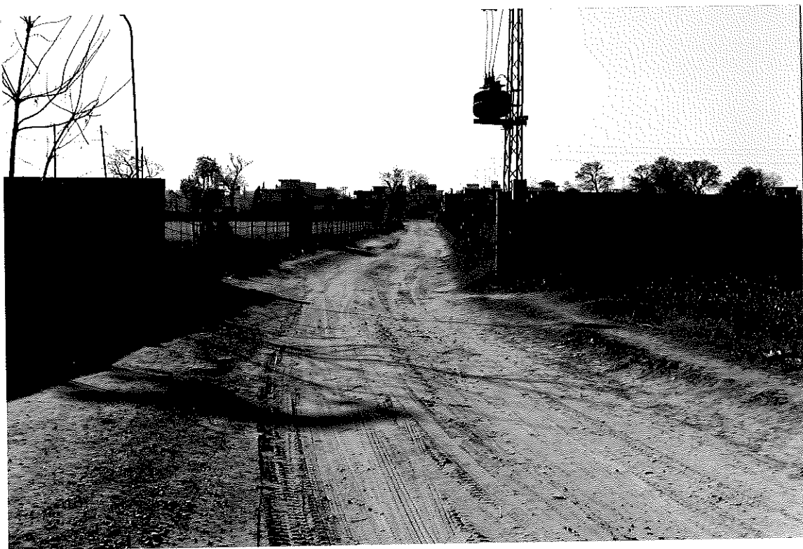
Photograph - 11: Humak-Jawa Road showing surface condition with gravel loss
